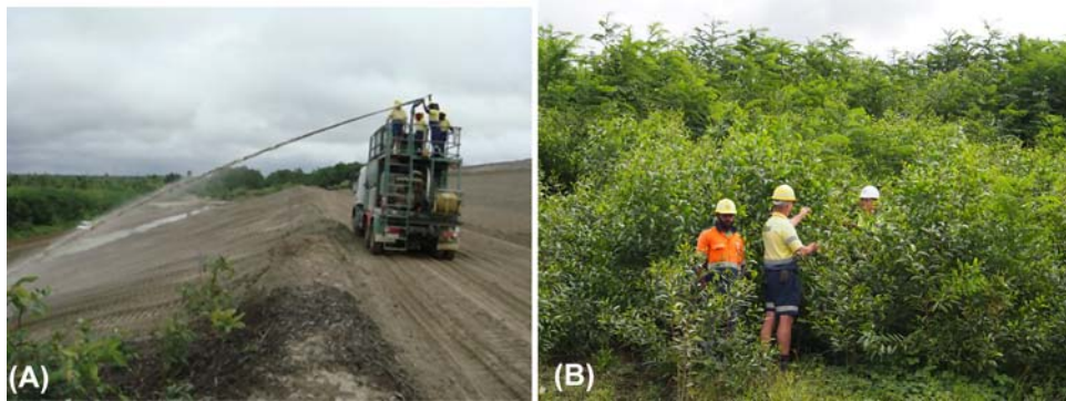
FIGURE 28.5 Representative photographs of OTML hydroseeding batter slopes (left) and resulting vegetation growth 18 months later (right).
